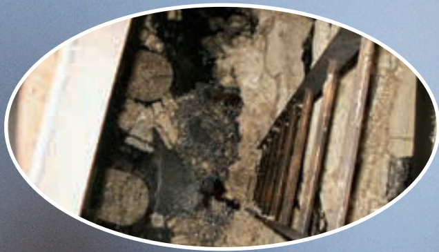
Waxy fuel in storage tank
